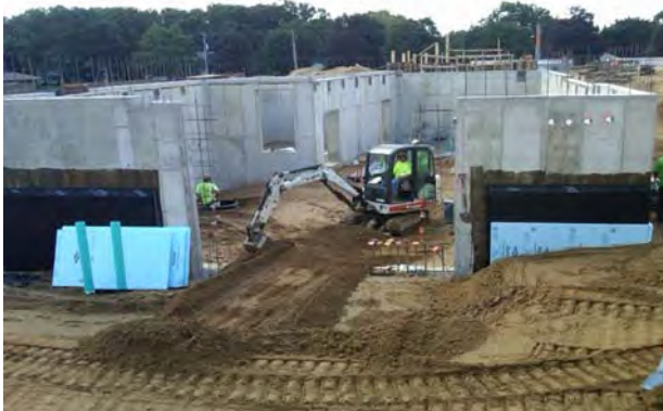
Excavation for the installation of acid waste lines
