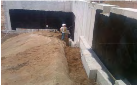
Dampproofing on Area C in process
