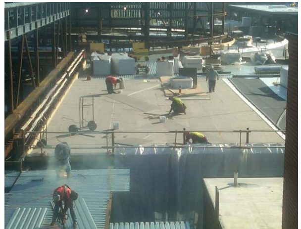
Roofing installation at Area B
