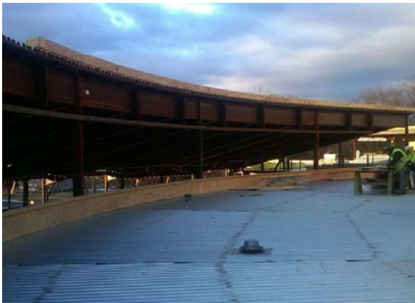
Roofing work at light monitors
