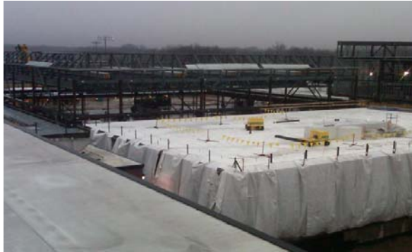
Area B roofing under way
