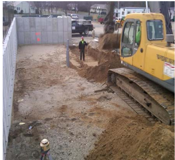
Excavation at generator room
