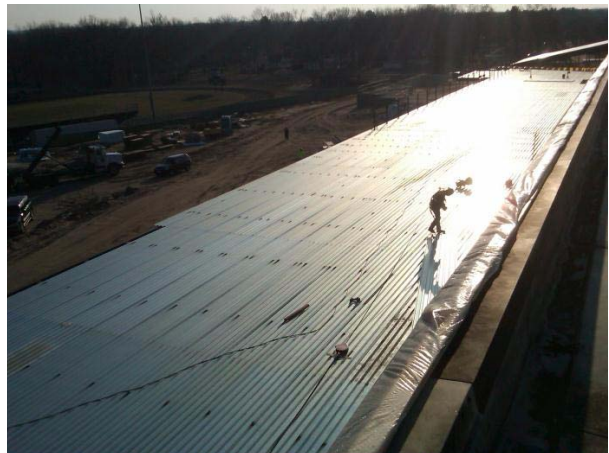
Roofing over locker rooms
