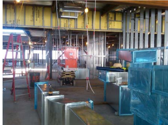
Ductwork installation under way
