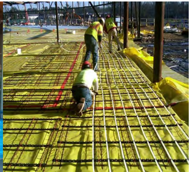
Radiant piping installation
