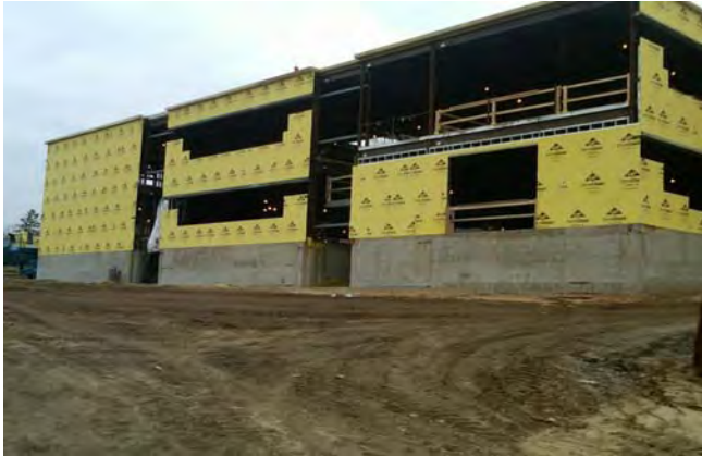
Exterior sheathing at Area C
