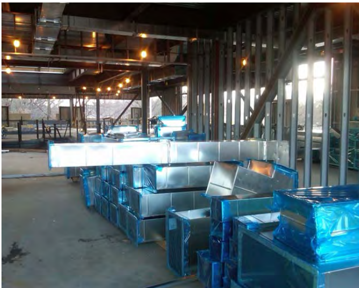
Ductwork received on site, ready for installation
