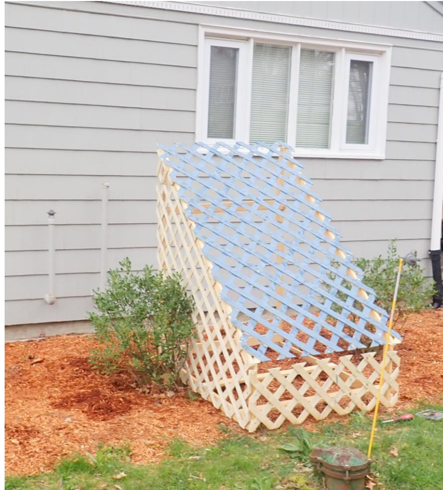
Ground-Mount Solar Panels
